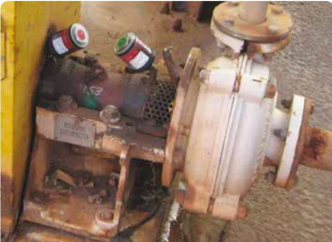
Application Horizontal slurry pump labyrinth seals Lubricator perma FUTURA Installation kit Direct mount
