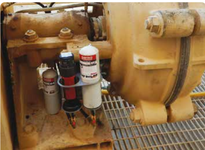
Application Slurry pump labyrinth seals & bearings Lubricator perma STAR VARIO L250 Installation kit K230C
